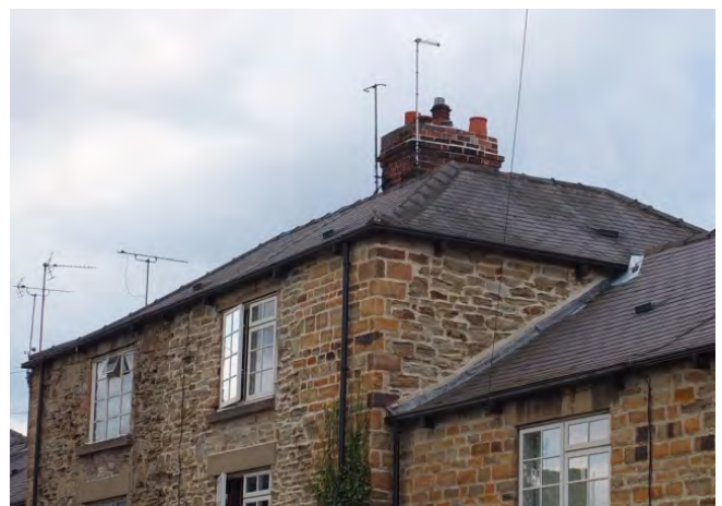
Photo 5 – hipped Welsh slate roof (Station Row)
