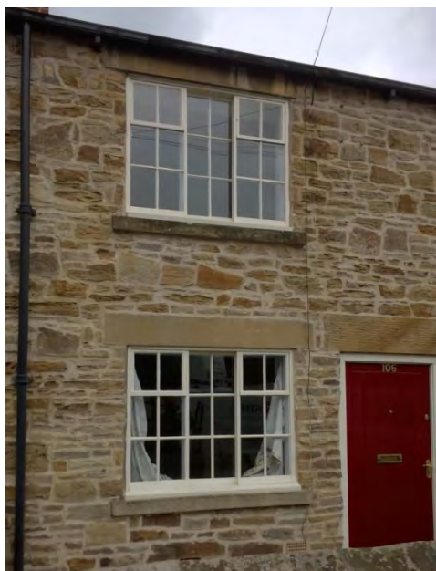
Photos 26 and 27 – Yorkshire sash replacement windows (Reform Row) and metal casement (Station Row)
