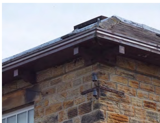
Photo 10 – Wooden box section gutter supported by wooden corbels
