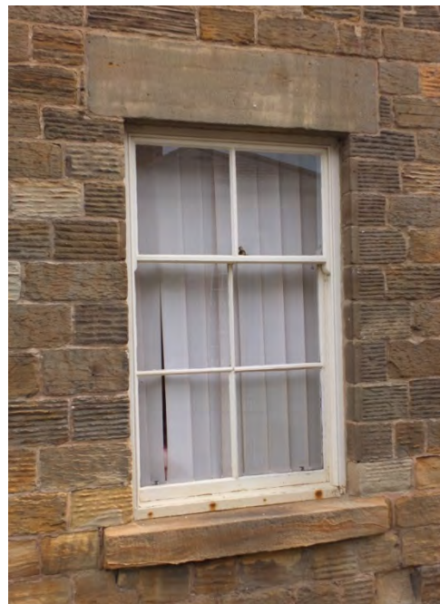
Photos 24 and 25 – timber sliding sash windows of different types, with narrow glazing bars
