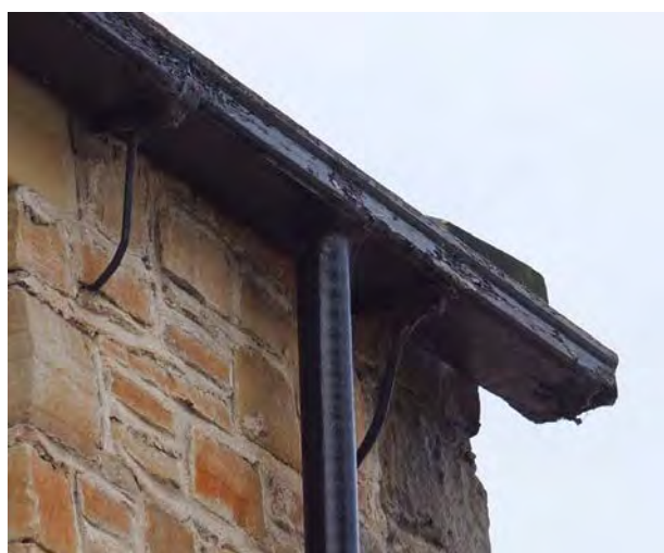
Photo 9 – Wooden box section gutter supported by rise and fall metal spikes
