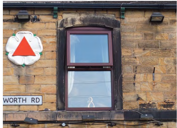
Photo 16 – carved stone head, jams and sill band to window opening (Market pub)
