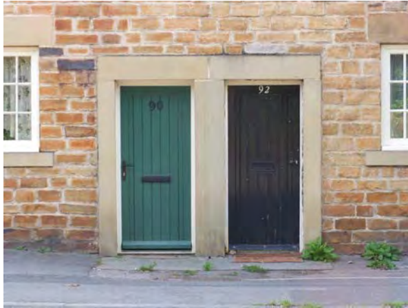
Photo 15 – simple monolithic jams and heads to doorways (Meadow Row)
